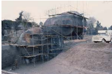
p) Immersion exhibits under construction
